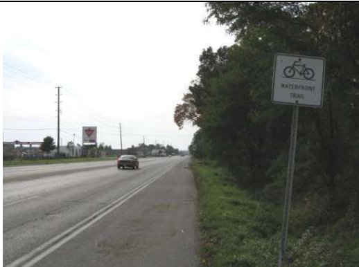
A paved-shoulder, signed cycling route on Elgin Street that is part of the Waterfront Trail.
