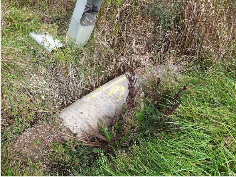
Culvert beneath unopened road allowance, Section 2
