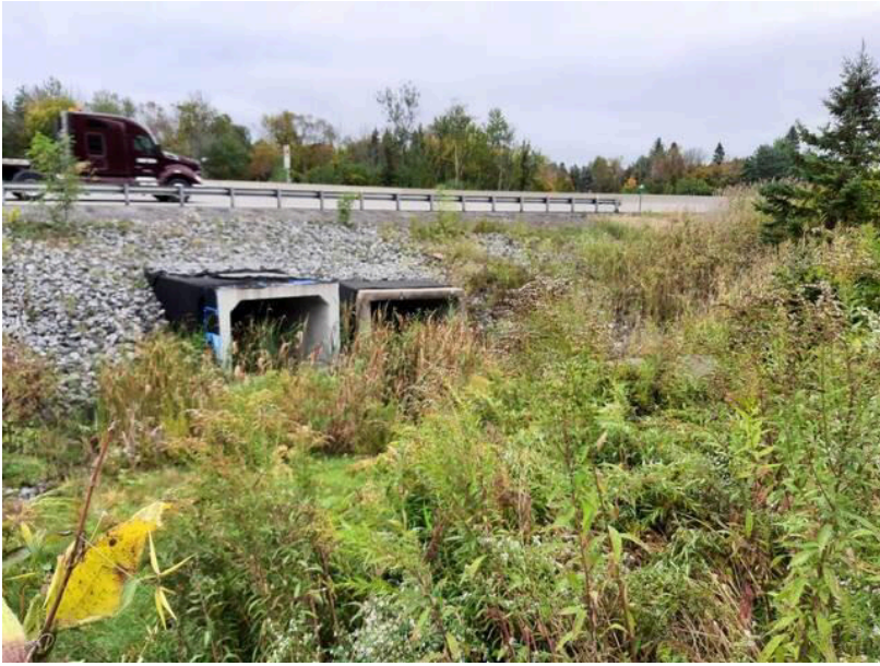
Box culvert under 401 at WCC#1a (WL#1)
