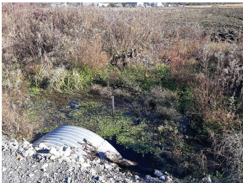
View toward the east at WCC#2
